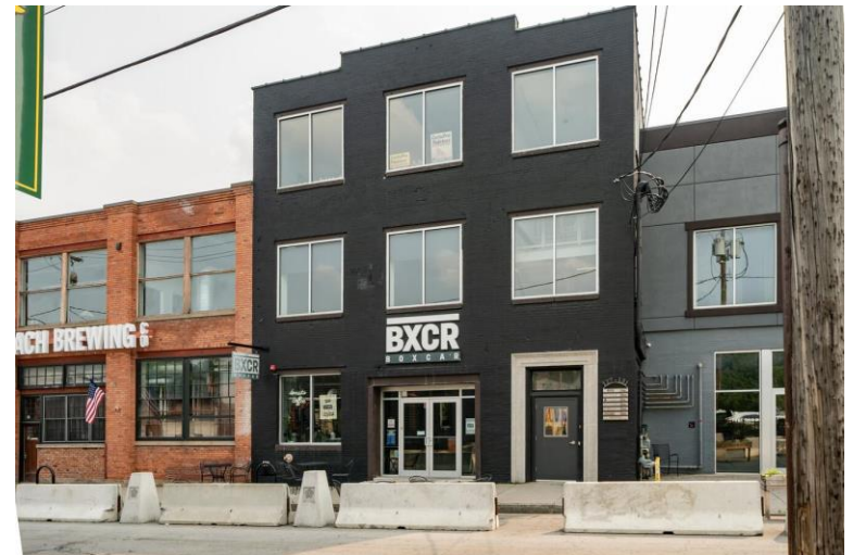
The interior & exterior condition
